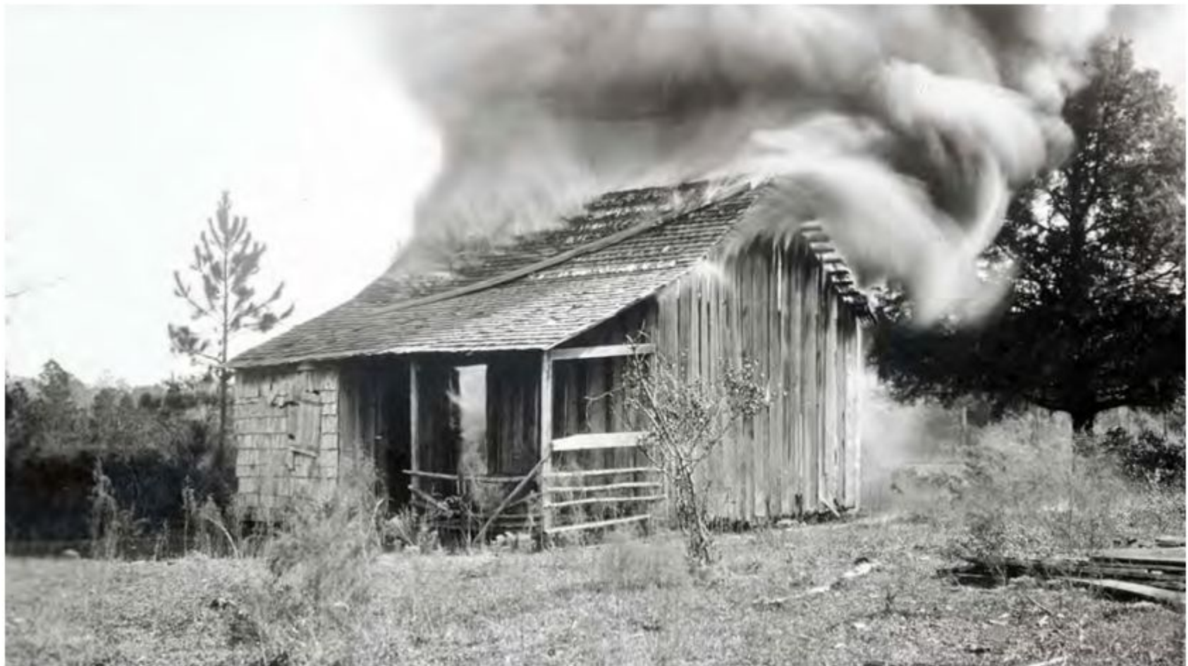
Rosewood Cabin Burning
